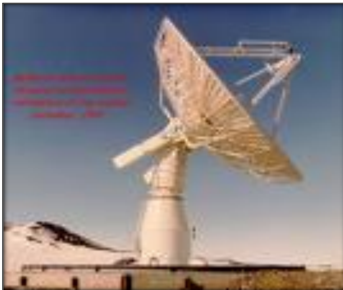
Figure 4: 10-meter antenna at McMurdo Station before the radome installation.
